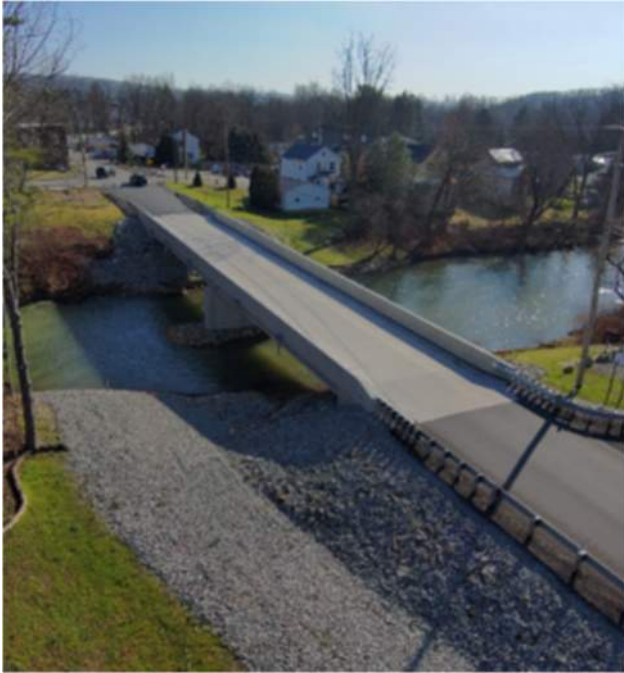
SR 3016 over Two Lick Creek
